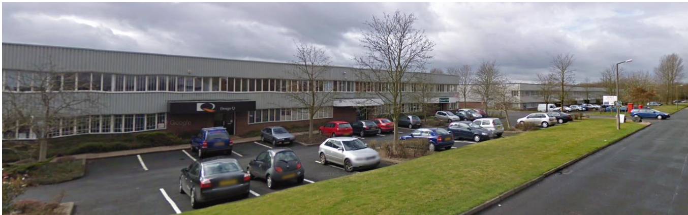
Photo from google (2009) looking at site from the North along Hemming Road
